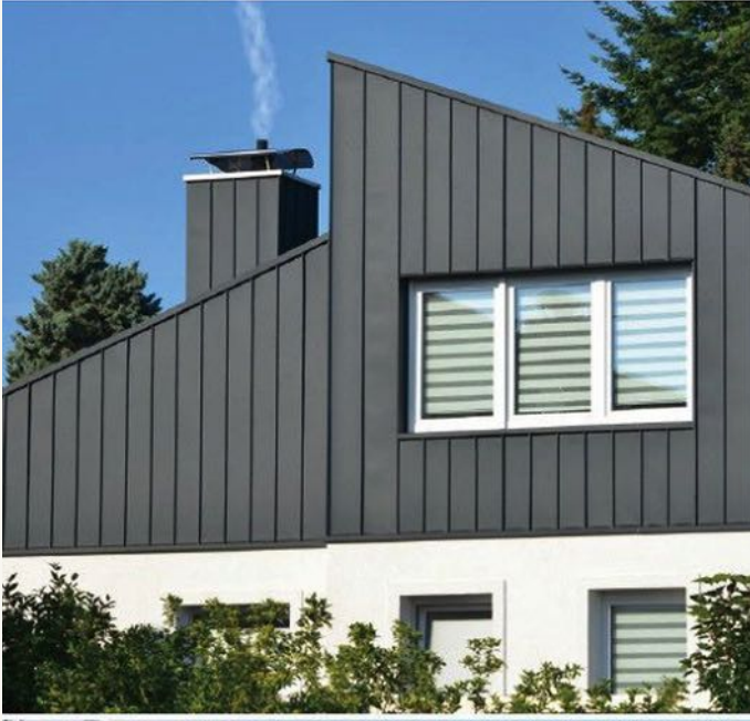
Building exterior materials
